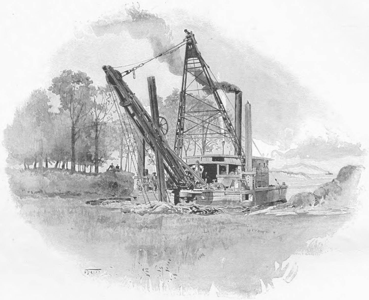
THE FIRST DREDGE, AUGUST, 1891.
