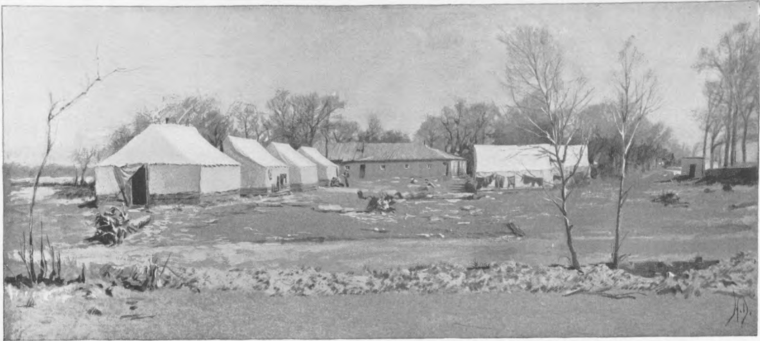
THE SITE OF ELECTRICITY BUILDING.
