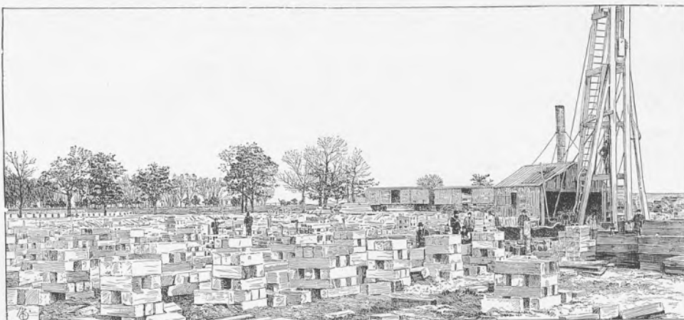
THE FOUNDATIONS OF THE GOVERNMENT BUILDING.
