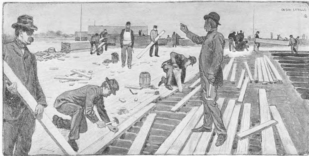
FLOOR LAYING, MANUFACTURES BUILDING.
