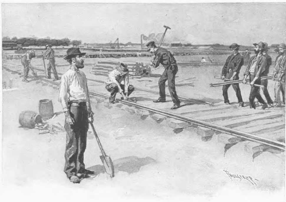
LAYING CONSTRUCTION TRACKS.
