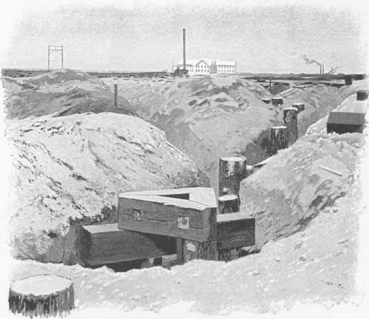
THE FOUNDATION OF ADMINISTRATION BUILDING, SEPTEMBER, 1891.
