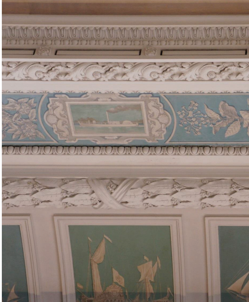
4.22 Millet, 'Fulton's "Clermont," the First Steamboat on the Hudson, 1807,' ceiling frame, north side, Call Room.
